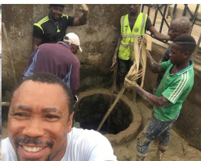
Refurbishing the well
